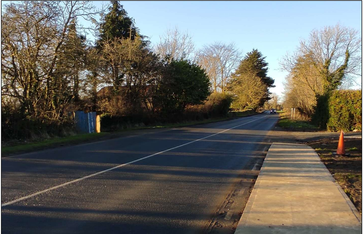
Figure 3 | Existing Footpath Termination at Carnew Road (facing west) at CH 500
